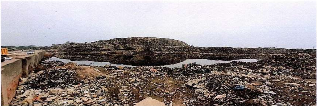
Plate-5: Photograph showing the leachate generated at legacy waste dump site.
