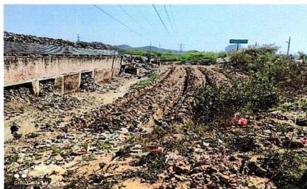
Plate-3 : Temporary boundary wall without plantation.
